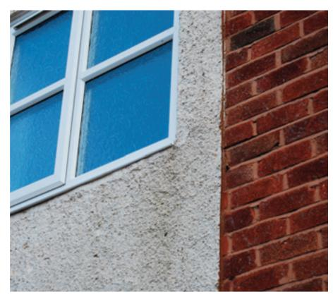
This photo shows a bathroom window recently installed which was clearly measured incorrectly on height, writes Don Waterworth.
