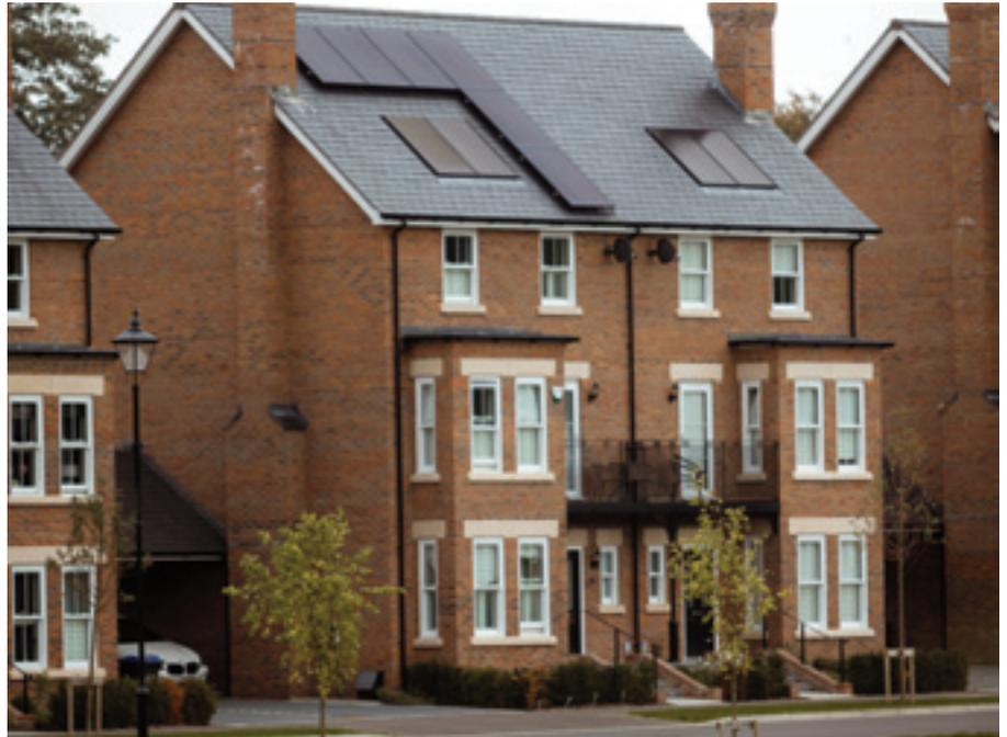
high-end homes that blend traditionally inspired detailing with stylish and comfortable modern design. Quickslide supplied vertical sliders in white PVC-U with a single astragal bar in both the top and bottom sash. No sash horns were requested,
