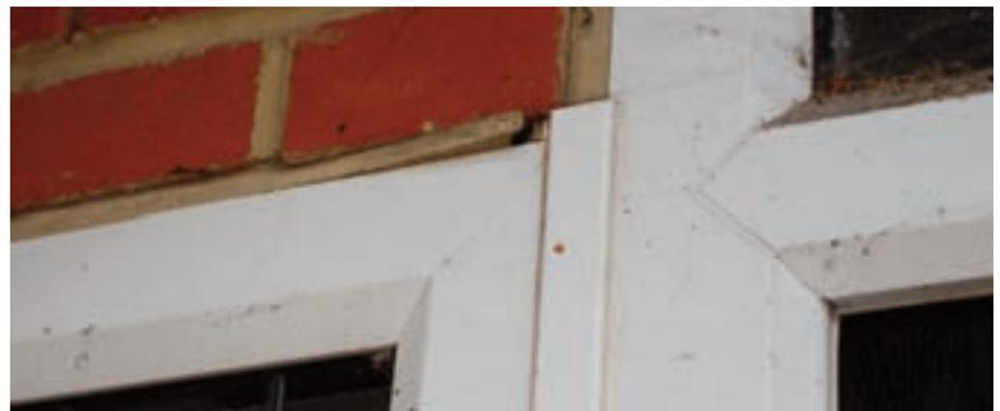
once the mortar fillet has cured, you will need to return to site and apply a low modulus silicone seal to the abutment joint between the mortar and the window or door frame.
