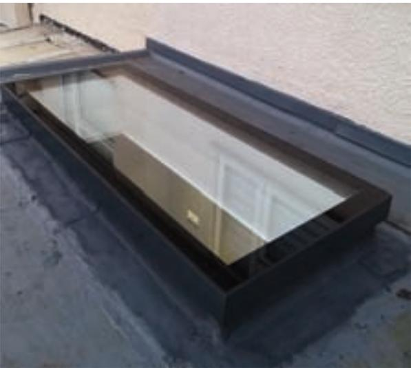
The 1000 x 2500mm standard stock clear glass Infinity fixed rooflight required much less space than a roof lantern, while ensuring the benefits of natural light flooded into the footprint of the building, giving the whole area a well lit, welcoming feel throughout of day.
