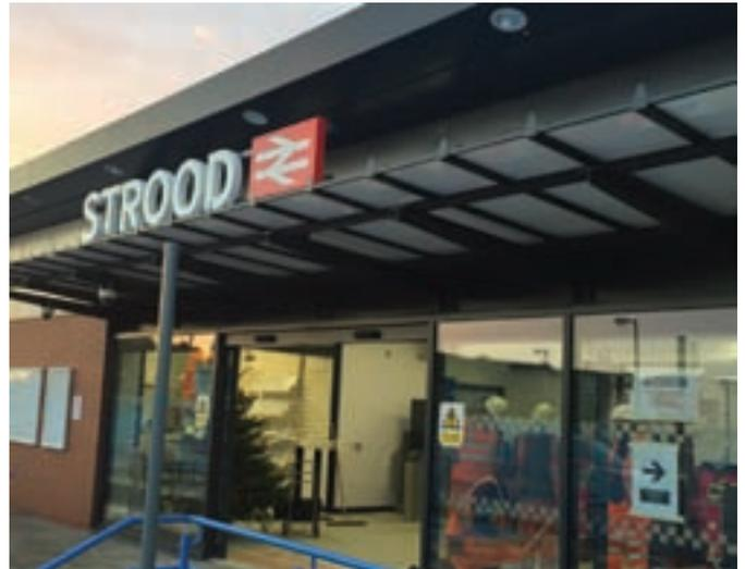
By choosing a remote access TD68 Thermal Door option with a built-in electric strike, staff at the railway station have full remote access control. The door can be locked internally and externally with a key to ensure it is secure on the outside. It can still be opened in an emergency from the inside using a standard panic door exit device.
